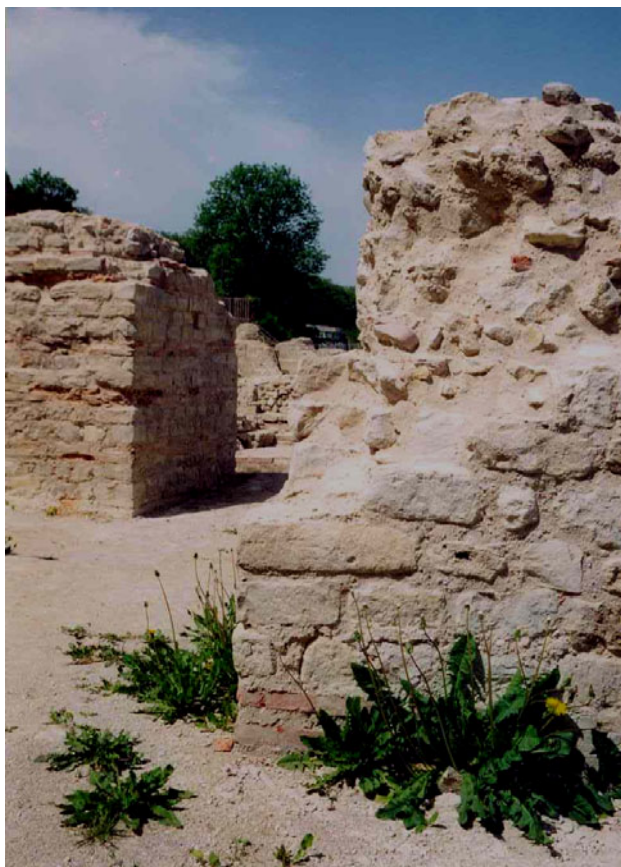
Fig. 3. Pillars of the sub-construction of the Roman Theatre at Mainz, showing the inhomogeneous environment of mortar and recommending TLD measurements for environmental dose rate determination.
