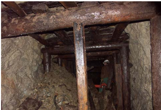
Fig. 2. Wooden casings in the gold mine in Złoty Stok
